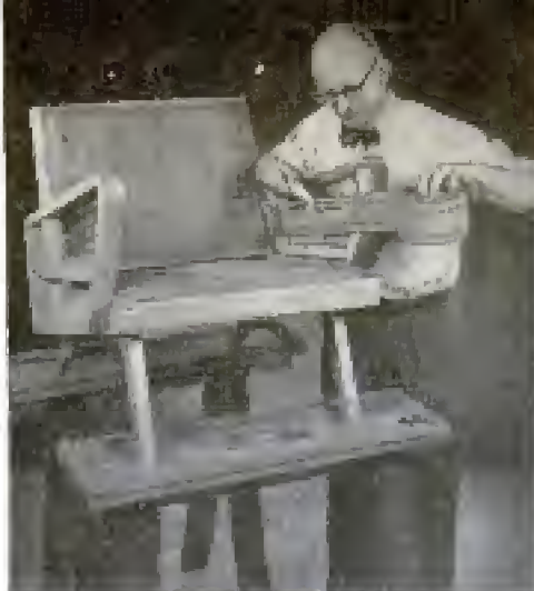
Above, chair arms are covered on inside with furniture webbing. Back and seat have already been covered with burlap. Below, photo shows chair padded with foam rubber and ready for fabric cover. Cotton is used to pad arms on outside
